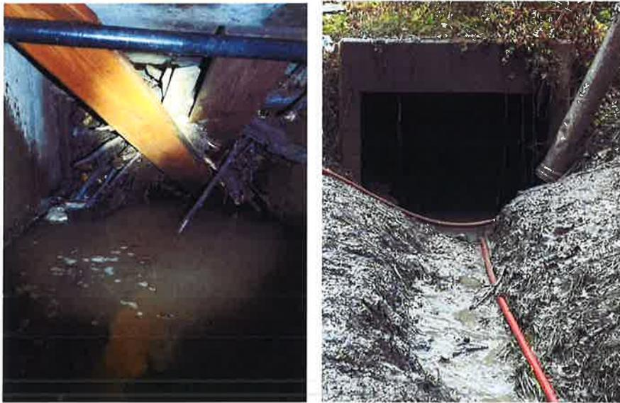
The pictures show an example of why developing an ordinance and educating the public about stormwater drains is important. This is a stormwater culvert that Ace recently cleaned out and it was filled with debris. When storm drains become blocked like this, it can lead to flooding and standing water. These kind of materials should not be in a storm drain.
